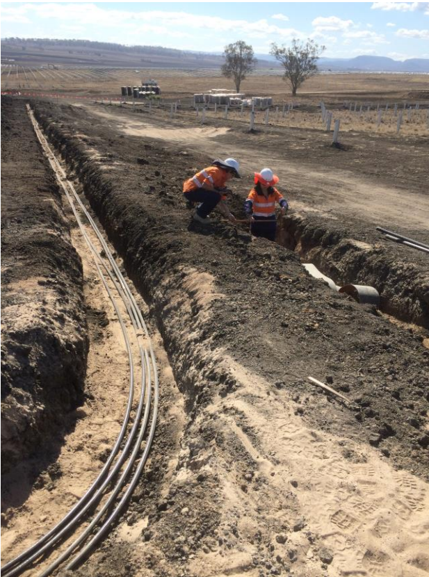
On-site inspections – checking trenches and cables for correct installation
