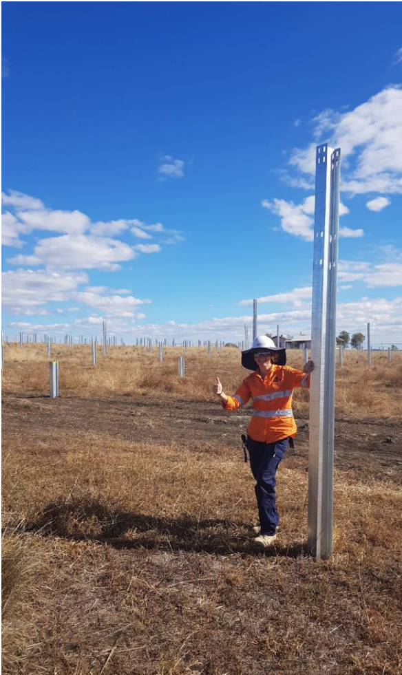
Sarah Haskmann, Project Officer, Energy and Sustainability When piling doesn't go to plan – this is what happens when you hit a rock during the pile drive!
