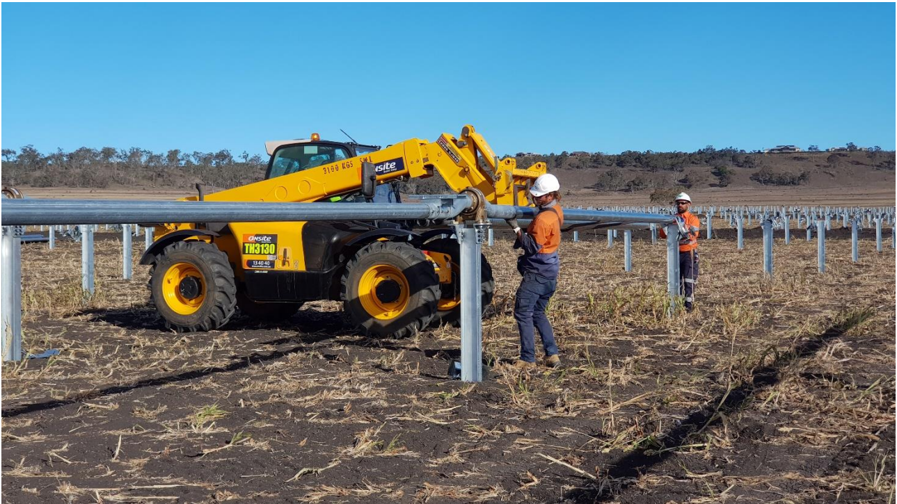
Torque tube installation
