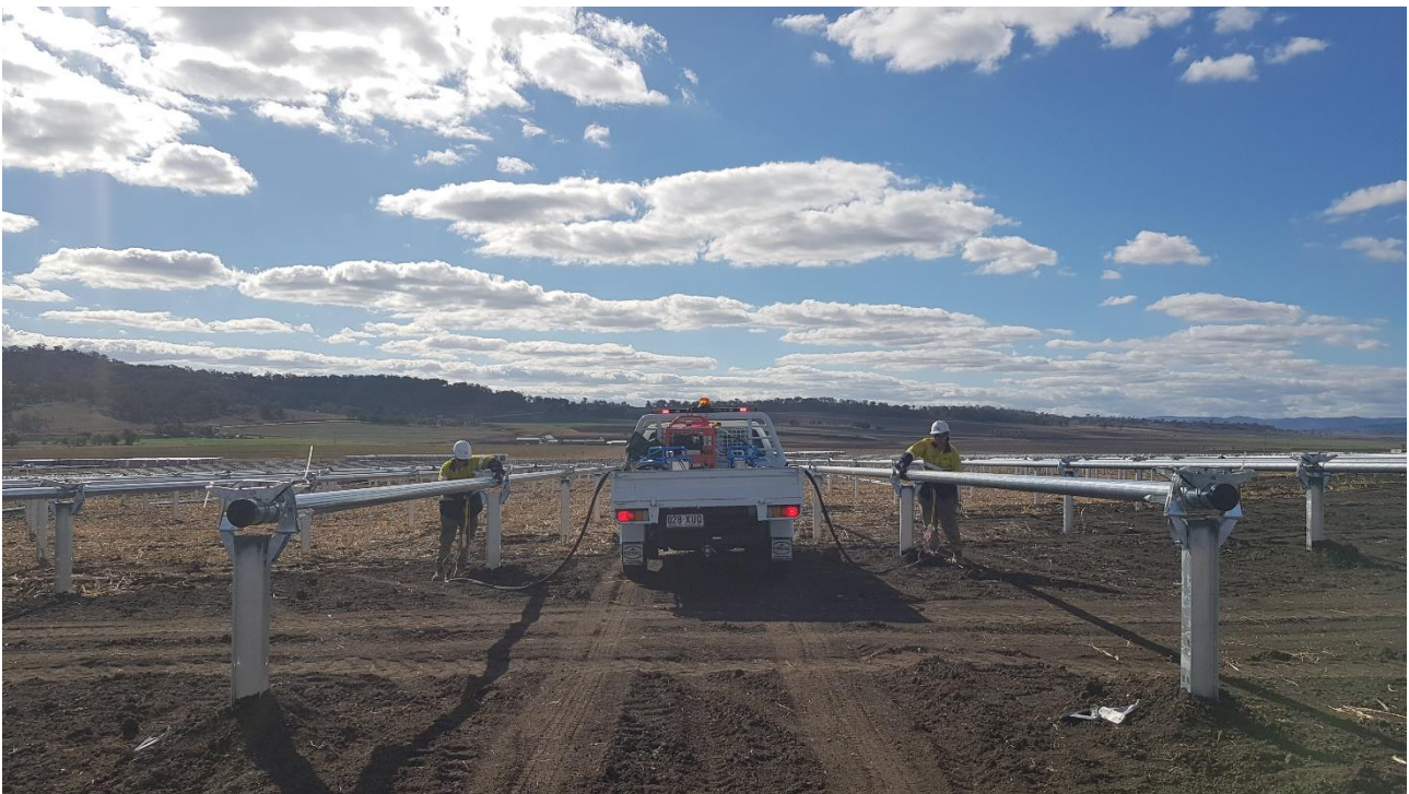
Torque tube fastening
