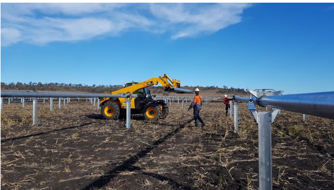
Torque tube installation
