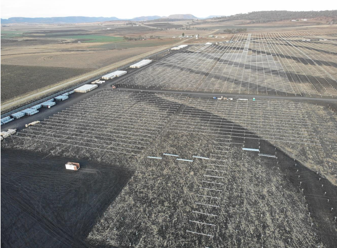
Torque tube installation aerial
