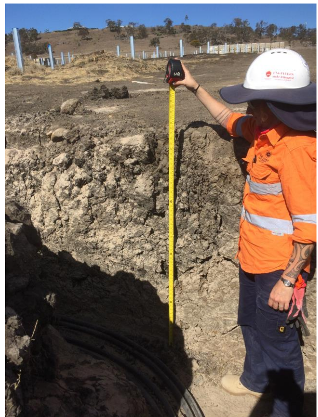
On-site inspections – checking trenches and cables for correct installation
