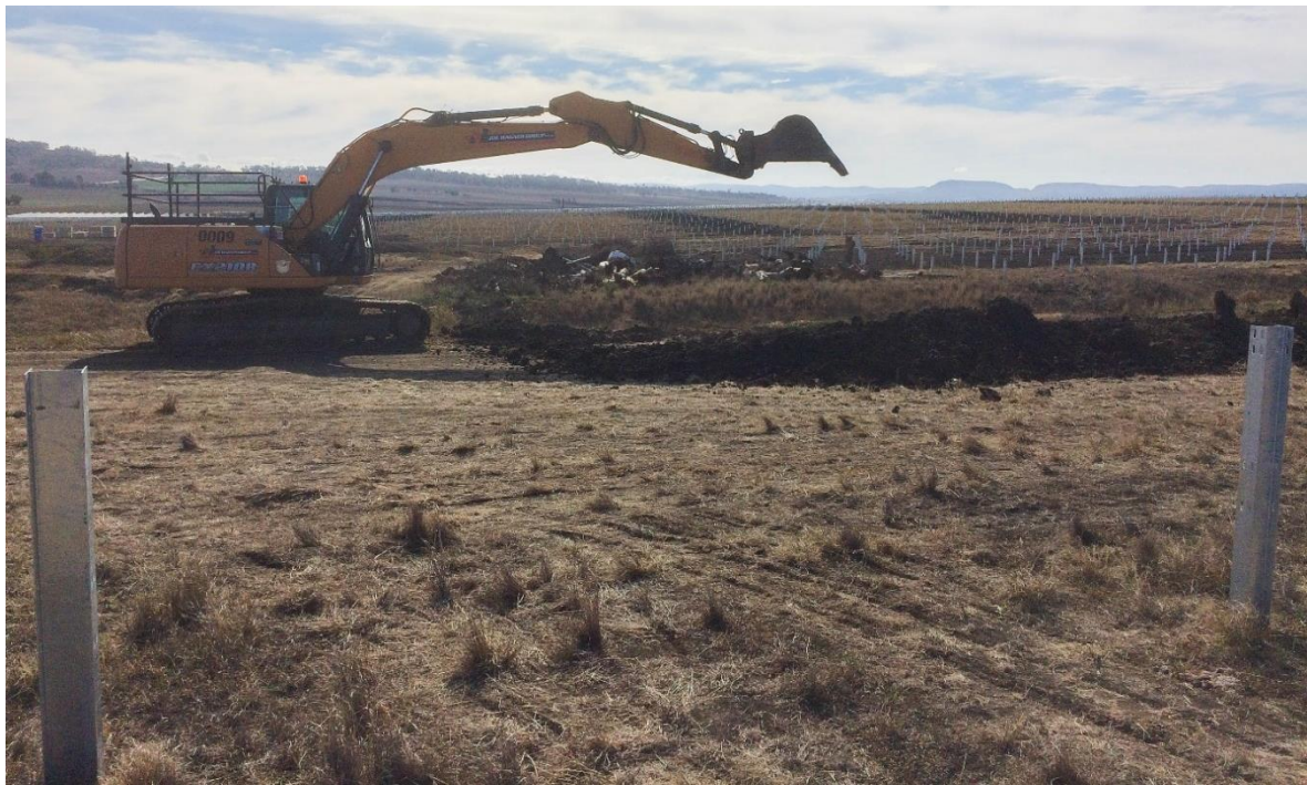
Excavator digging a DC trench – trenches are often 100's of metres long and dug perfectly straight
