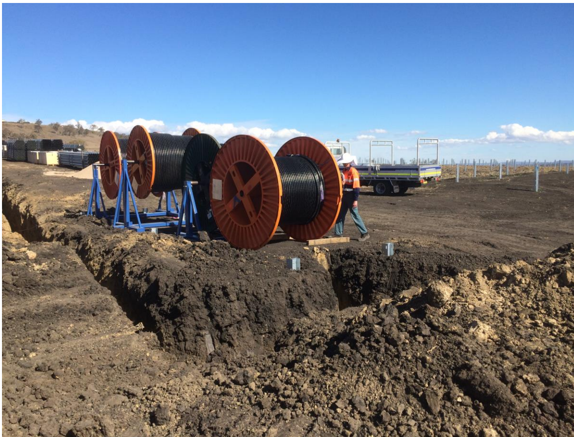
DC cable drums – staged for cable installation
