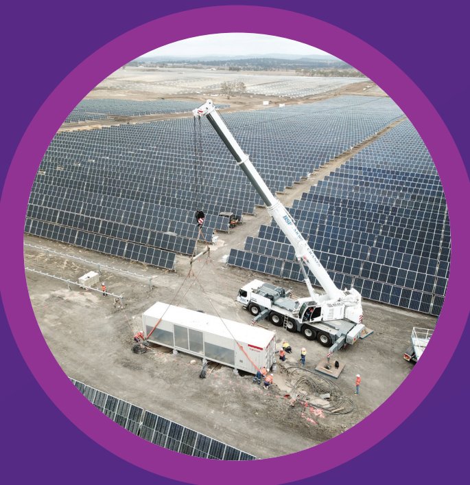
Lifting & mounting of Power Conversion Units Late Sep 2019–late Oct 2019
