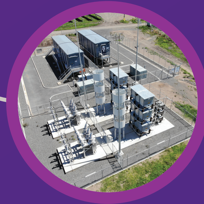
Harmonic Filter & Switchyard construction Mid Jul 2019–end May 2020
