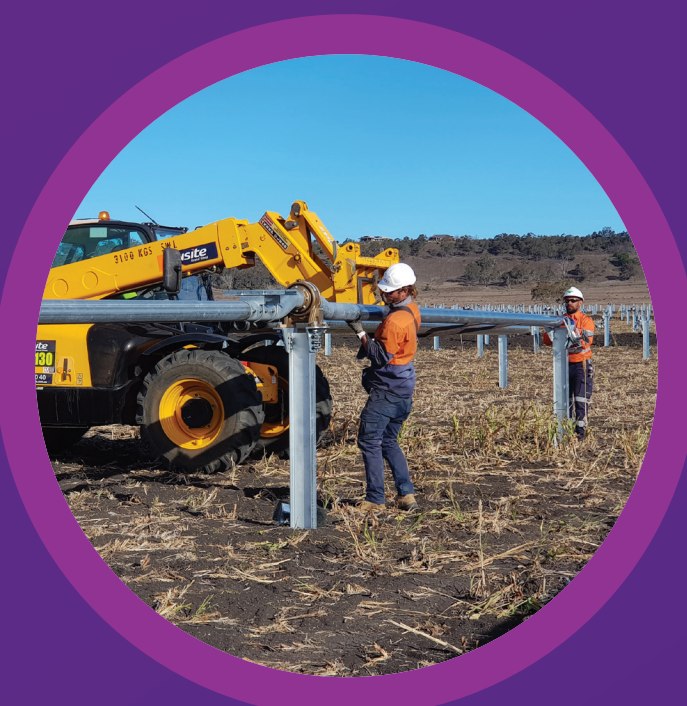
Installation of tracker torque tubes & motors Late May 2019–late Oct 2019
