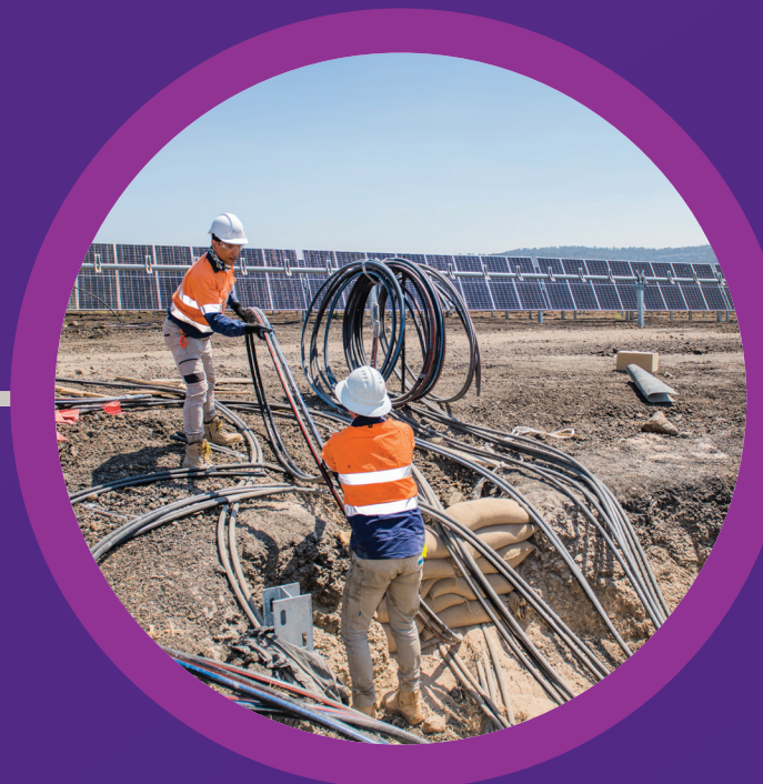
Installation of underground cable Late Jun 2019–late Sep 2019
