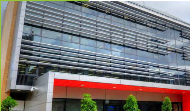
Below: Sun shades at Prentice Building to protect the northern facade from direct sunlight.
