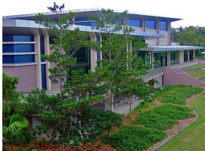
Figure 6: UQ Centre Eastern Facade
